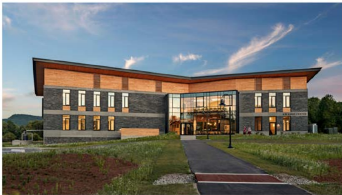
Figure 4. The R.W. Kern Center at Hampshire College is a certified Living Building at Hampshire College [21].
